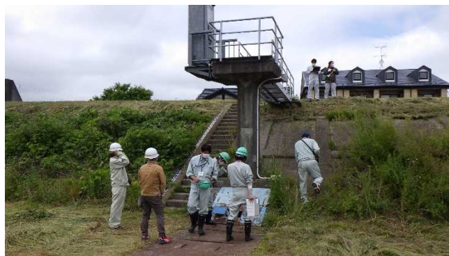
▲樋門樋管点検
