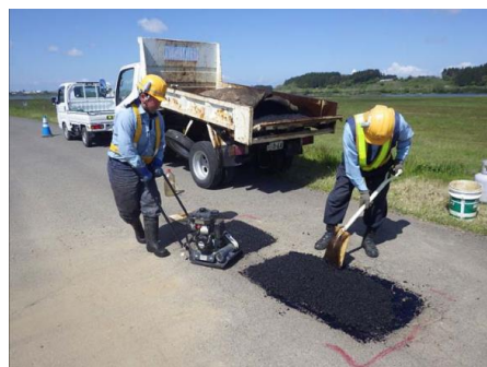
堤防天端の補修状況
