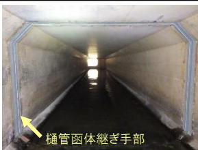
樋管管体継ぎ手補修
