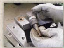
▲ Tightening the bolt with care to avoid over-tightening.
