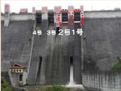
▲ Crest Gate No. 1 and 2 water seal rubber replacement in progress!
