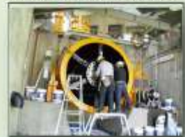
<Repairing a release valve>
