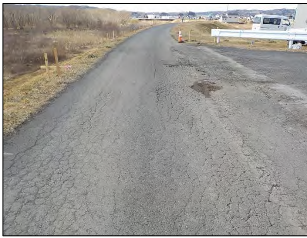
堤防天端舗装(浅水川付近)【打換え】前
