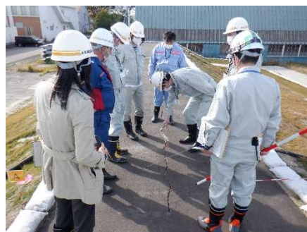
▲ 堤防天端の亀裂の深さ計測
