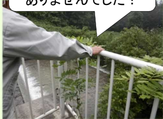
▲入間砂防堰堤
