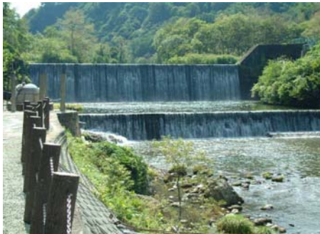
▲肘折砂防えん堤
