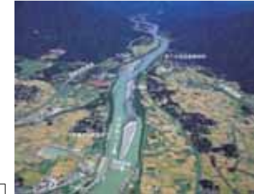
渡場床固工～馬下頭首工付近
