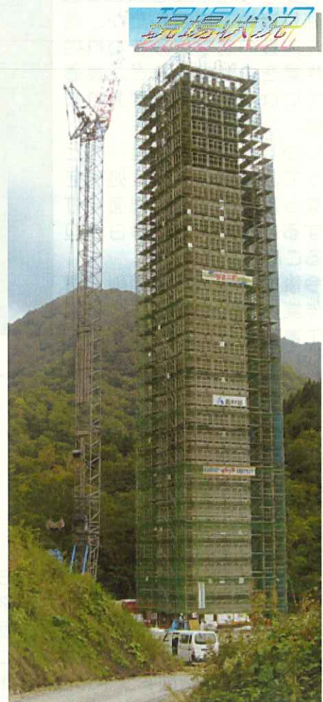
(P2橋脚施工状況)
