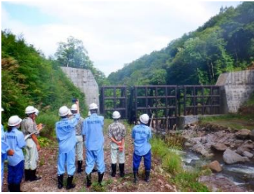
▲塩の川第7砂防堰堤
