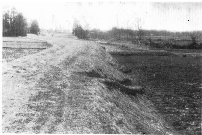
24 押切堤防 (S48.3)
