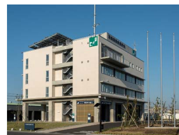
[石巻港湾合同庁舎(国施設)]
